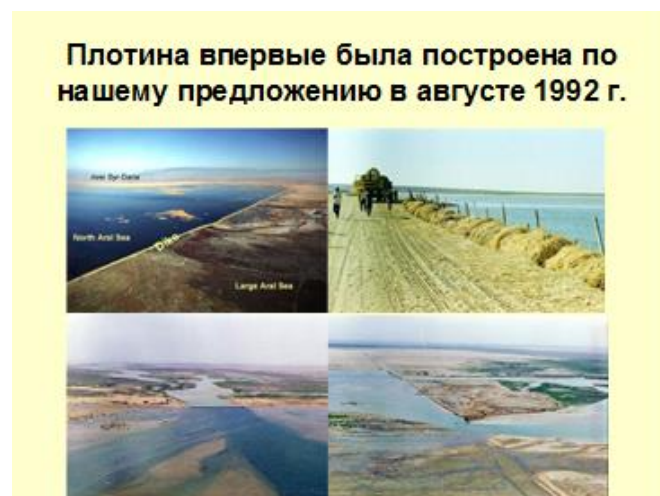
Figure 7: Building of the dam
