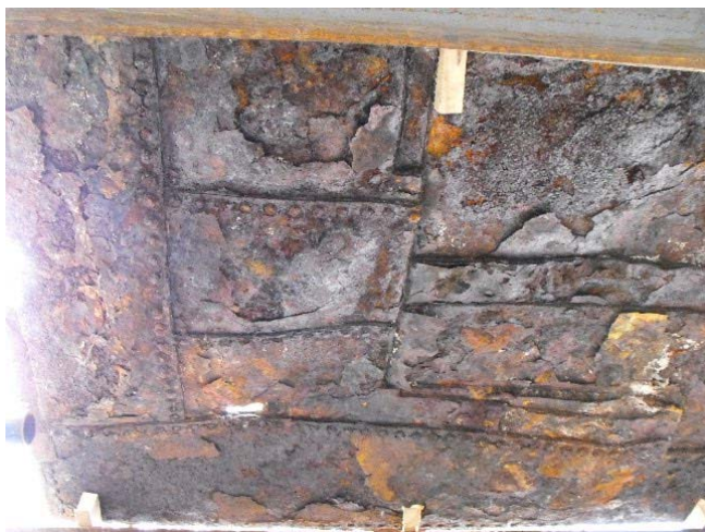
Fig. 8. The underside of the salt pan shows the patchwork of iron plates which had been riveted, and later welded, in place to mend holes caused by corrosion in the iron pan
