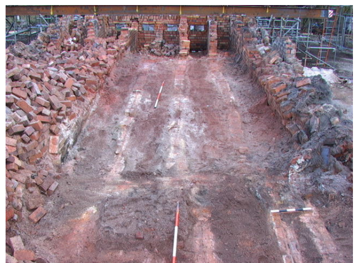
Fig. 7. Dismantling the flues which ran beneath Salt Pan 5. The view is from the Stove House end, looking back towards the stoke holes. This pan had been built to burn coal, but was converted to burn oil
