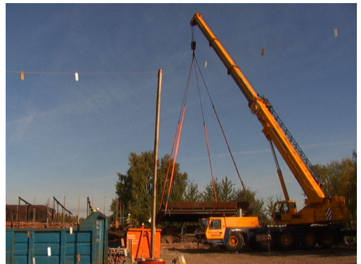
Fig. 6. Lifting Salt Pan 5 from off the furnace base
